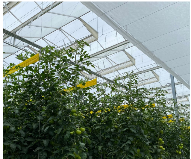
Figure 23. Accordion-style exclusion screens covering roof peak vents.
